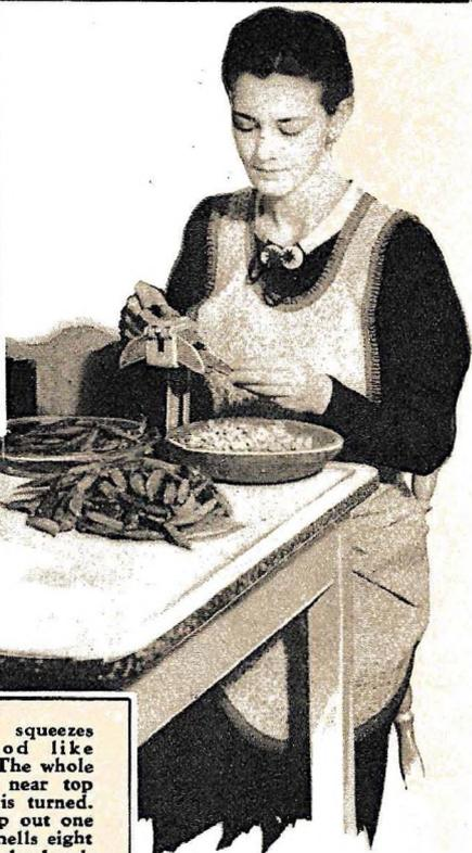
**PEA-SHELLER** squeezes peas from pod like clothes-wringer. The whole pod is inserted near top and the handle is turned. Empty pods drop out one chute. Device shells eight times faster than by hand.
