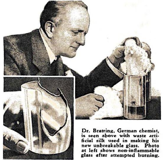
Dr. Brating, German chemist, is seen above with waste artificial silk used in making his new unbreakable glass. Photo at left shows non-inflammable glass after attempted burning.
