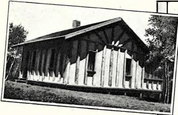
Here is a side view of the completed cabin, showing the sunburst roof supports and rear door from the kitchen.
