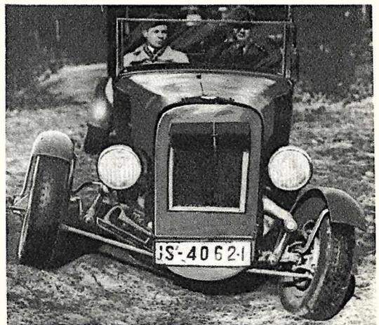
Swaying or tilting when driving around curves or over bumpy roads is claimed to be eliminated with this "curve-balancer." Metal elbows allow independent movement of the wheels.
